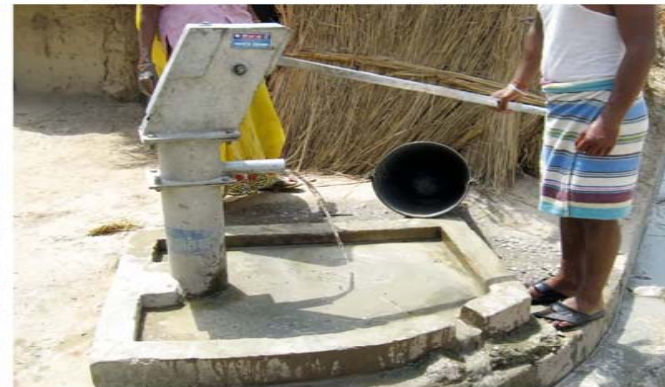
BLOCK: KOTWALI CODE:203 VILLAGE:HASAN ALI PUR HEERA LOCATION:BALBEER KE PASS
